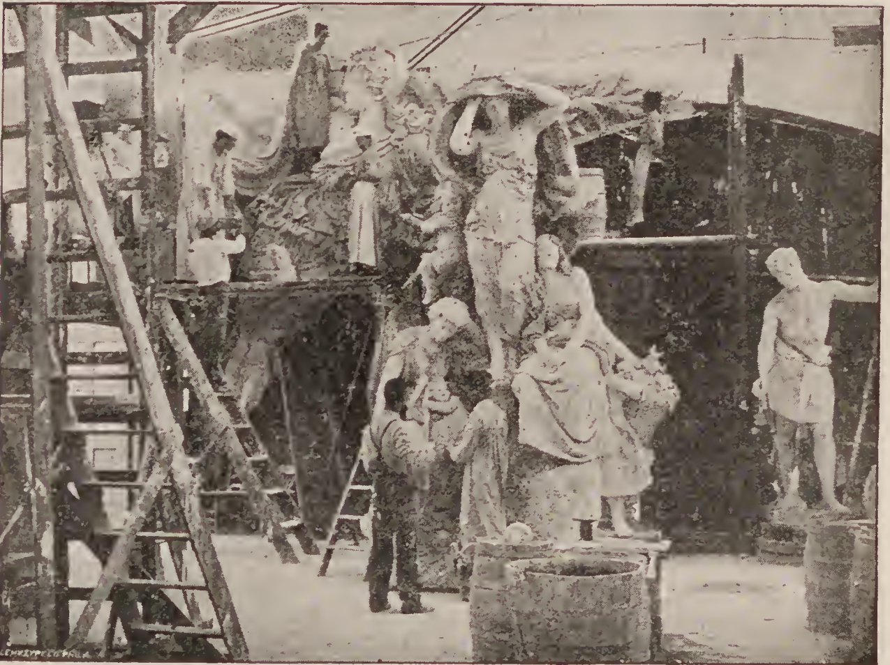
LORADO TAFT'S STUDIO IN HORTICULTURAL HALL. (Showing Sculpture for the Building Under Way.)
